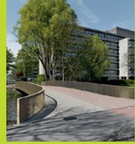
A prefab composite FiberCore bicycle bridge has a lifespan of more than a hundred years and is maintenance-free and vandal-proof.
