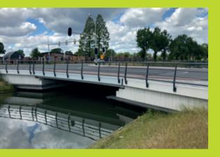
FiberCore traffic bridges are a sustainable solution. They are lightweight and therefore easy to install; guickly and with minimal disruption. Due to their low-maintenance nature, they are worry-free. Only the wearing surface – depending on the circumstances – needs to be replaced or updated after a while.
