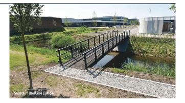
compared to traditional materials are its high strength, low energy requirement during construction, low maintenance requirement and long service life, with no rot or corrosion. As a result, the bridge material is expected to last for at least 100 years.
