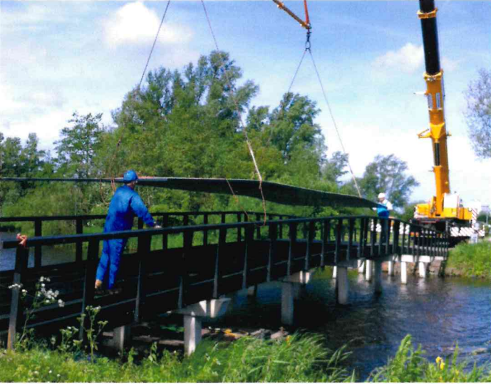
Installation of a 15x4m InfraCore® Inside deck.
