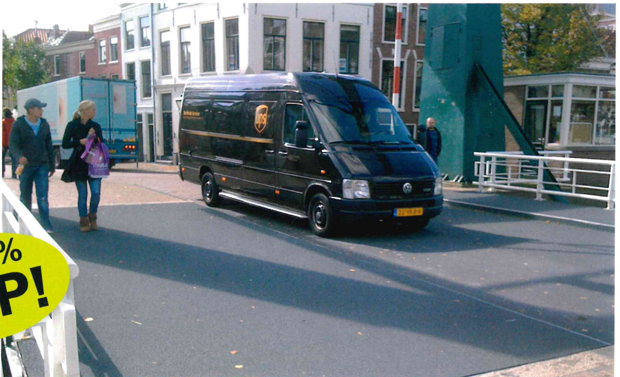
Bridge deck refurbishment with a watertight InfraCore® Inside deck.
