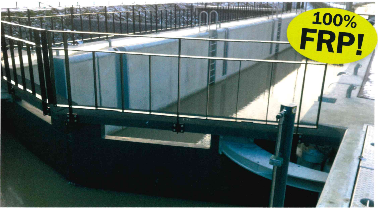
InfraCore ® Inside FRP lock gates in Kanaal Erica-Ter Apel.
