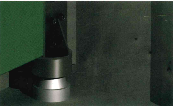
Connection lock gate to lower hinge.
