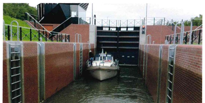
Inside the lock chamber of the Kanaal Erica-Ter Apel.
