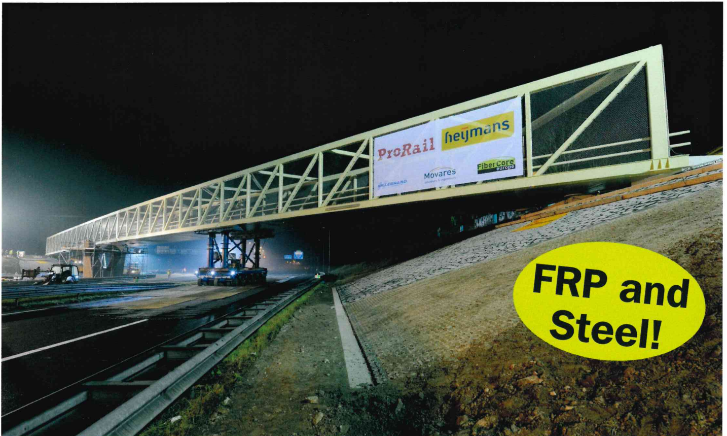
An FRP-steel hybrid bridge halfway during installation across the A27 motorway near Utrecht, the Netherlands. Design and construction of InfraCore® Inside-deck: FiberCore Europe.
