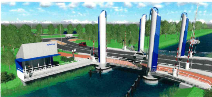
The lifting cables of this hybrid lifting bridge are attached to a steel beam integrally connected to the InfraCore® Inside deck.
