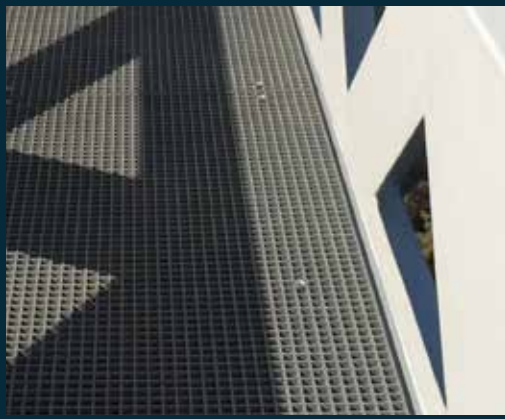
Maintenance-free composite open grating floor, equipped with wear-resistant surface layer.
