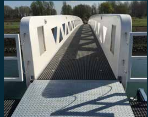
Pivot point and sliding support for tidal circumstances.
