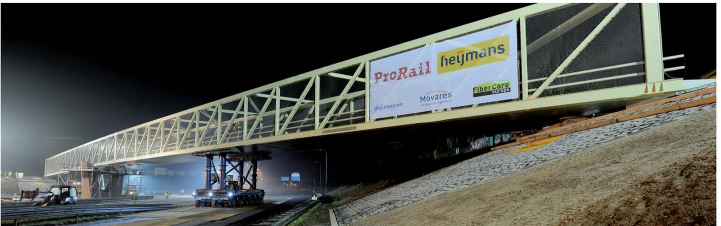
In the deck of this 142m viaduct the thermal expansion properties of the InfraCore® Inside deck were modified. This allowed the deck to be integrally connected with the steel trusses.
