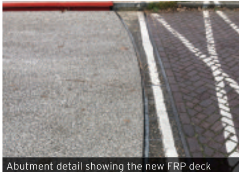
Abutment detail showing the new FRP deck
